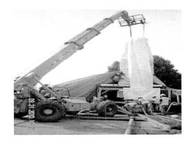
**<u>Project Description</u>**: Rehabilitation of 18,569 feet of sewer ranging in size from 10-inch diameter to 8'x4'6" box sewer by cured-in-place pipe method and spray-on lining systems; rehabilitation of an inverted siphon; rehabilitation of 63 structures by the spray-on lining system; raising of two manholes; abandoning 290 feet of 20-inch pipe; cleaning 500 feet of 8'x4'6" box sewer.
