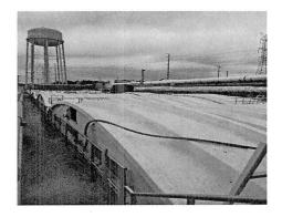
**Project Description:** The remaining old gravity concentration tanks will be converted to the Waste Activated Sludge Stripping to Remove Internal Phosphorus (WASSTRIP®) process to aid in the release of phosphorus which will be recovered from the pre-digestion centrate by the existing Ostara process.
