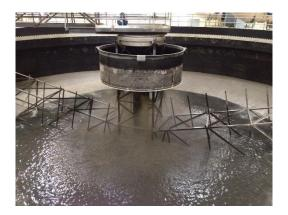
**Pro ect Description:** This project will convert two of the new gravity concentration tanks (GCTs) into fermenters and install a pumping station to pump the fermentate directly into the West Side primary effluent conduit feeding the secondary aeration batteries. This project will also install a gas detection system for the new gravity concentration tank building.
