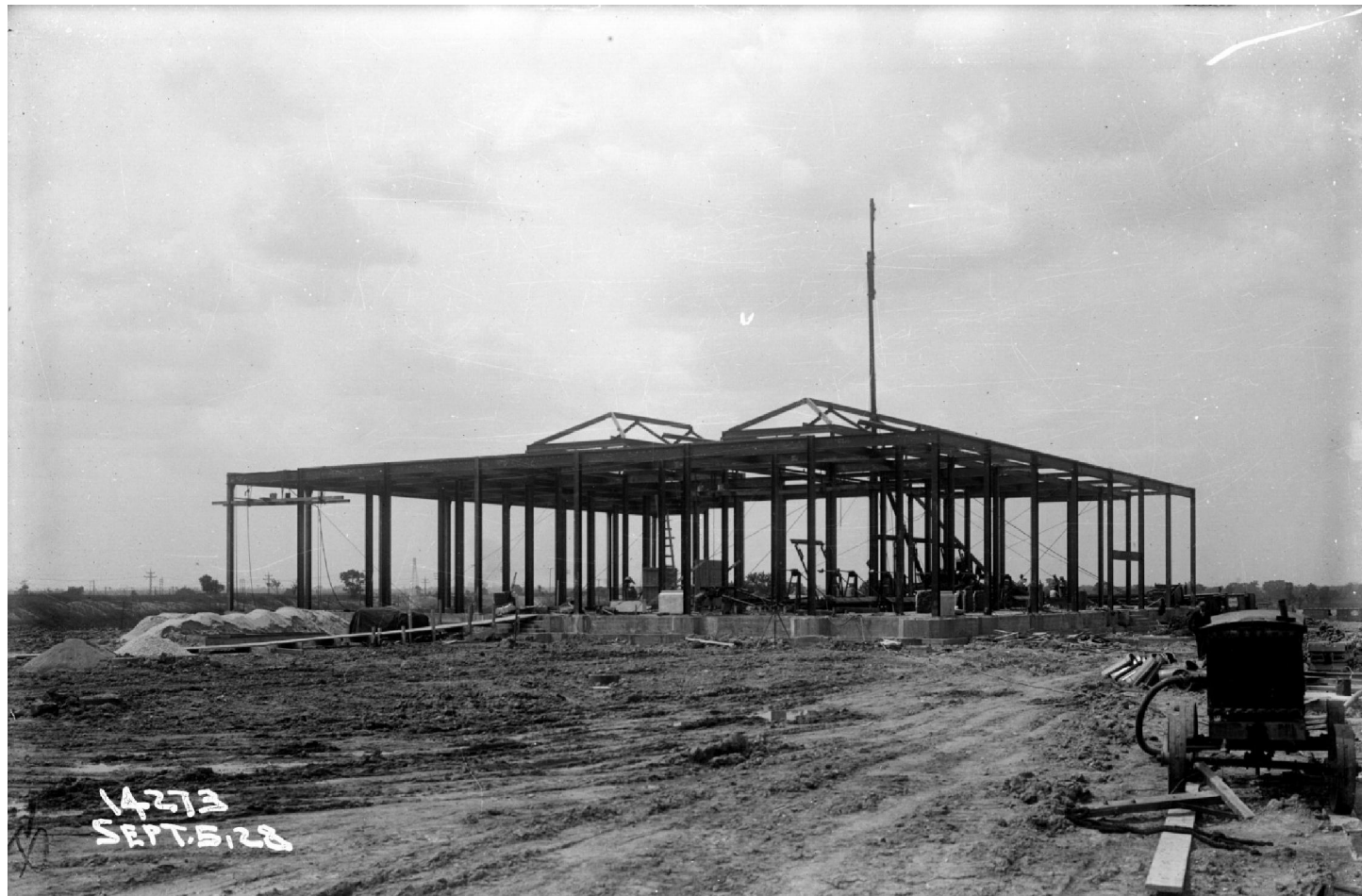
Fine Screens Building Under Construction
