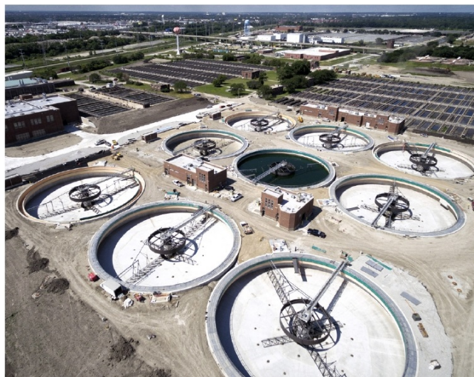
The District is constructing new primary settling tanks and aerated grit tanks, support facilities, service tunnels, and conduits at the Stickney Water Reclamation Plant. This will replace tanks, produce renewable energy, increase and improve grit removal, protect downstream piping and equipment, increase water recycling and reduce odors.
