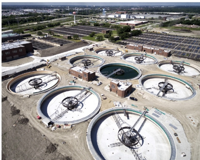
The District is constructing new primary settling tanks and aerated grit tanks, support facilities, service tunnels, and conduits at the Stickney Water Reclamation Plant. This will replace tanks, produce renewable energy, increase and improve grit removal, protect downstream piping and equipment, increase water recycling and reduce odors.
