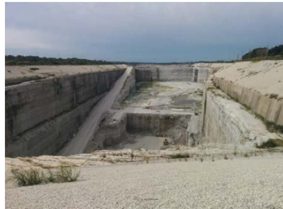
McCook Reservoir Stage 1 mining operations, at the lowest level of the reservoir.
