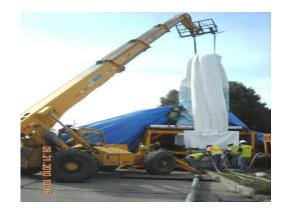
**Project Description:** This project includes the rehabilitation of 18,569 feet of sewer ranging in size from 10-inch diameter to 8'x4'6" box sewer by the cured-in-place pipe method and the spray-on lining system; rehabilitation of an inverted siphon; rehabilitation of 63 structures by the spray-on lining system; raising of two manholes; abandoning 290 feet of 20-inch pipe; cleaning 500 feet of 8'x4'6" box sewer; construction of an access manhole.
