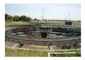
**Project Description:** Group A: Painting of the final tanks at the Stickney WRP. Recoat the interior rake arm and center column portions, which are constructed of ferrous metal, on 22 final settling tanks.
