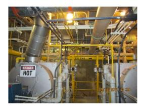
**Project Description:** Provide four hot water boilers, three heat exchangers, hot water circulating pumps, and piping for the digester complex and administrative building. Provide an electrical room in the digester complex and relocate motor control centers into the new electrical room. Also included is the removal of the existing boiler systems in the administrative building and digester complex.
