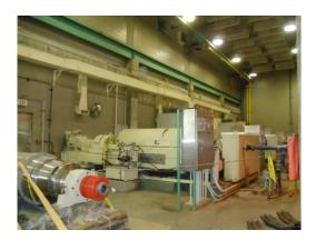
Project Description: Rebuild four centrifuge rotating assemblies and gearboxes at the Egan WRP.
