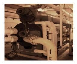
**Project Description:** Furnish, deliver, and install generator section tubes for Chiller 1 at the Egan WRP.
