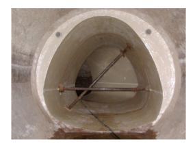
**Project Description:** The work consists of rehabilitating approximately 32,800 feet of intercepting sewer with sizes ranging from 10" in diameter to 7'0"x7'0" semi-elliptic concrete pipe using the cured-in-place pipe lining method and/or the channeline lining method, rehabilitating 80 manholes by the spray-on lining system, rebuilding and raising 12 manholes, constructing one manhole, and making control structure modifications.
