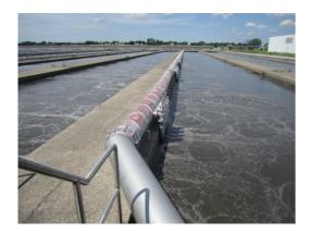
**Project Description:** Install stainless steel guard rails around the existing aeration tanks and preliminary tanks for safety reasons to meet OSHA regulations. In addition, the concrete will be repaired as required to anchor the railings around the tanks.
