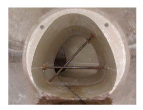
**Project Description:** The rehabilitation of 6,590 feet of 40"x62" egg shaped sewer by the cured-in-place lining method and/or the channel lining process and the rehabilitation of eight manholes by spray-on products. The spot repair of 20 feet of 27-inch diameter sewer and the rehabilitation of 347 feet of 27" sewer pipe.
