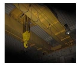
**Project Description:** Rehabilitate and recondition eight overhead cranes. Resolve deficiencies found during Contract 07-932-11 on the North and South Pump House and service bays, wheel gate gantry, and the dewatering and discharge valve chamber cranes.
