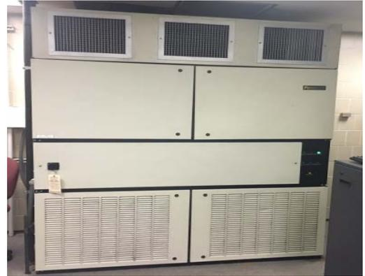
**Project Description:** Demolish and remove five air conditioning systems and furnish, deliver, and install replacement systems. The systems include the Administration Building computer room HVAC and supplemental cooling, the Administration Building control room cooling, the digester control room cooling, and the Tunnel and Reservoir Plan control room cooling.
