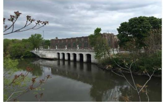
**Project Description:** Provide grouted fiberglass fiber reinforced plastic jackets around the existing concrete columns to protect columns from erosion. Repair underwater deteriorated concrete of the east wall and under the deck wall. Repair deteriorated concrete stairs and concrete deck. Restore balustrade and deck lighting.
