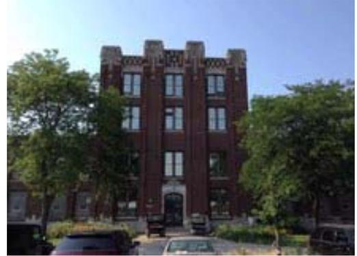
**Project Description:** This contract provides for the restoration of the Process Control Building at the O'Brien WRP. The scope of the project includes grinding and recaulking the capstones and limestone, tuckpointing the entire structure, removing and replacing the sealant on all the doors and windows, replacing all the windows and glass blocks, and removing and replacing the roof. This project is expected to have a life expectancy of over 20 years.
