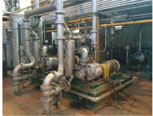
**Project Description:** Replace problematic equipment and install modern technology to ensure increased dependability of the vacuum pump priming systems at the 95th Street Pumping Station and reduce the risk of flooding during rain events. The installation will be performed by District pipefitters.
