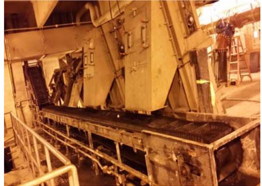
**Project Description:** Demolish and remove existing sludge conveyor and furnish, deliver, and install an upgraded sludge concentration conveyor and washer compactor.
