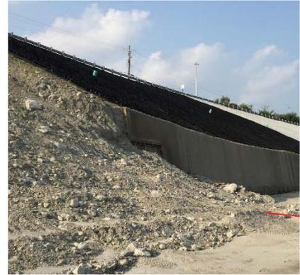
**Project Description:** The scope of work consists of constructing approximately 2,000 linear feet of a soil nail retaining wall along the western and southern sides as well as slope stabilization work around the entire perimeter of Expanded Stage 2 of the McCook Reservoir.
