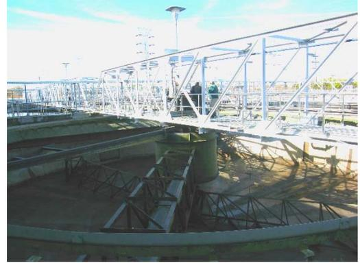
**Project Description:** The project will remove an existing steel and wood baffle plate in Final Settling Tank B-1. The contractor will also furnish and install circular, fiber reinforced, and plastic baffle plates and support framing under the bottoms of the influent wells in each of the converted final settling tanks.
