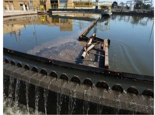
**Project Description:** Furnish, deliver, and install new clarifier drives on four final tanks and new mixers on one digester and one concentration tank. Refurbish and paint the structural steel members of six tanks. Refurbish two tanks per year.
