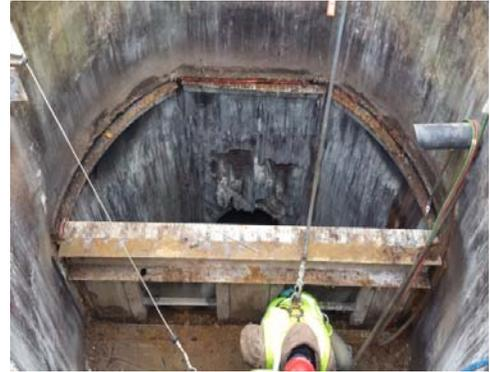
**Project Description:** The project consists of the rehabilitation of the following: Drop Shaft No. 5 by slip lining, 100 feet of 108-inch pipe by the cured-in-place pipe lining process, 75 feet of the drop shaft exit conduit by spray-on lining, and replacement of deteriorated appurtenances.
