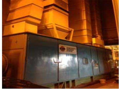
**Project Description:** Furnish, deliver, and install all equipment, materials, and appurtenances necessary to rehabilitate the three-megawatt digester gas turbine at the Stickney WRP central heat facility
