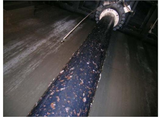
**Project Description:** This project will include the removal, rehabilitation, and installation of the hydraulic operator on the Tunnel and Reservoir Plan (TARP) Gate Structure 1 (GS-1) in the Calumet Service Area.
