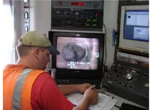
**Project Description:** To provide the District with sewer inspection services of varying methods including: video inspection, water jetter system television inspection, zoom camera inspection, laser profiling, multi-sensor inspection, and manhole and Tunnel and Reservoir Plan drop shaft inspection. The contractor will also be responsible for cleaning, disposal, and hourly video inspection services.
