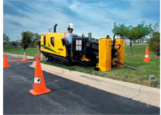
**Project Description:** This project consists of the installation of 2,000 linear feet of six-inch diameter pressure pipe by directional drilling and the installation of air relief, blow-off, and clean-out structures.
