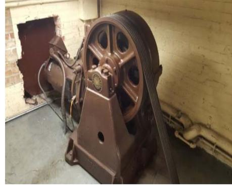
**Project Description:** Modernize two Main Office Building (MOB) elevators by replacing direct current motors on two machines with alternating current motors with variable frequency drives to ensure better, more reliable performance while achieving energy savings.
