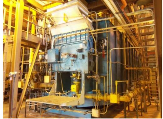
**Project Description:** This project will furnish, deliver, and install controls, programming, and other required appurtenances to provide a co-fire implementation of Boilers 3, 4, 5, and 7 using natural gas and digester gas through existing gas trains. Use of co-fire logic and technology shall enable full utilization of available digester gas produced at the plant. Controls for Boilers 1 and 2 will be upgraded as well.
