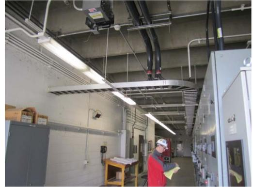
**Project Description:** Replacement of the medium voltage (13.2kV) switchgear and medium voltage feeder cables in D799 at the Stickney WRP.
