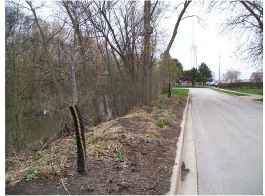
**Project Description:** The scope of this project involves stabilization of approximately 750 feet of Addison Creek adjacent to Fullerton Avenue in Northlake and 410 linear feet of streambank adjacent to 19th Avenue in the Village of North Riverside. Stabilization methods include the installation of native vegetation, a vegetated geogrid, turf reinforcing mat, and the placement of riprap.
