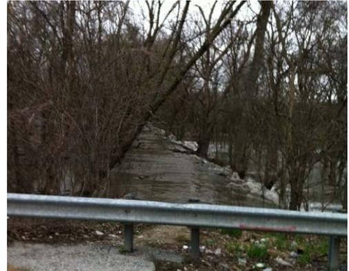
**Project Description:** The Lyons Levee is located on the east bank of the Des Plaines River and is approximately 4,000 feet long, beginning at Joliet Road at the upstream end and extending approximately 700 feet downstream of 47th Street. The scope of the project involves the restoration and improvement of the levee to a condition that will elevate the levee to modern design standards, provide flood protection, and prevent overtopping by events up to a 100-year design flood.
