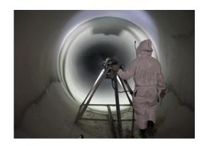
**<u>Project Description</u>**: This project consists of the rehabilitation of 810 feet of 6'x7' semi-elliptic cast-in-place concrete sewer and inlet/outlet structures. The Summit Conduit begins on the northwest side of the Des Plaines River and extends southeast under the Des Plaines River and the Stevenson Expressway to the northwest side of the Chicago Sanitary and Ship Canal.
