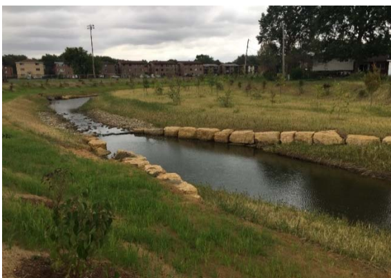
Streambank stabilization along Tinley Creek in Crestwood.
