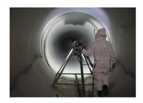
**Project Description:** This project consists of the rehabilitation of 810 feet of 6'x7' semi-elliptic cast-in-place concrete sewer and inlet and outlet structures. The Summit Conduit begins on the northwest side of the Des Plaines River and extends southeast under the Des Plaines River and the Stevenson Expressway to the northwest side of the Chicago Sanitary and Ship Canal.
