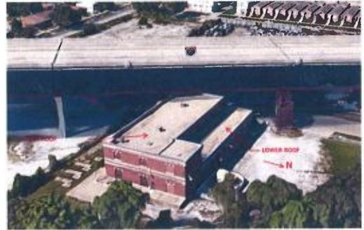
**Project Description:** Furnish labor, material and equipment required to replace water-damaged gypsum roof panels and repair or reinforce corroded structural steel members at the upper and lower roof levels. Replace the roof membrane and perform miscellaneous tuck-pointing and masonry work to eliminate water infiltration.
