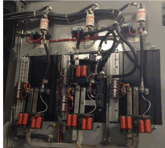
**Project Description** Furnish and deliver replacement excitation control equipment for the North Branch Pumping Station (NBPS) and the Racine Avenue Pumping Station (RAPS) main sewage pump synchronous motors. Four new pump motor exciter control systems will be installed at both the NBPS and the RAPS. Installation will be performed by District trades under the direction of an excitation control manufacturer representative and the resident engineer.
