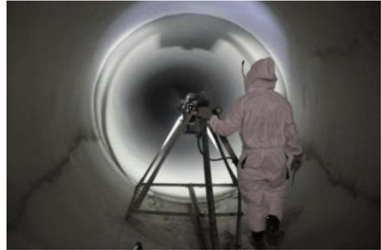
**Project Description** This project consists of the rehabilitation of 810 feet of six feet by seven feet semi-elliptic cast-in-place concrete sewer and inlet and outlet structures. The Summit Conduit begins on the northwest side of the Des Plaines River and extends southeast under the Des Plaines River and the Stevenson Expressway to the northwest side of the Chicago Sanitary and Ship Canal.
