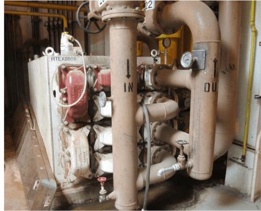
**Project Description** Removal of sludge heating boiler systems and installation of steam-to-hot water heat exchanger systems at the Digester Complex. Installation of steam and condensate piping with supports for the new system. Replacement of four sludge heat exchangers in Cluster 1 and replacement of tubes and gaskets for sludge heat exchangers in Cluster 2. Re-purposing of old compressor building for electrical equipment.
