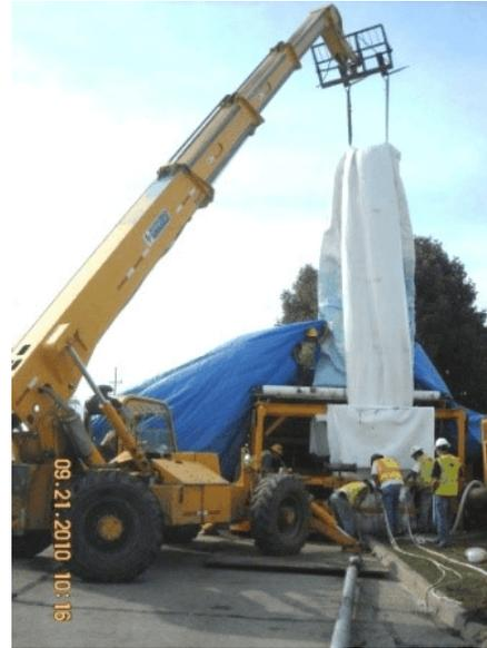
**Project Description** Project consists of rehabilitating 2,902 feet of 48-inch diameter sewer and 11,902 feet of 69-inch diameter sewer by cured-in-place pipe lining and/or the slip lining method, rehabilitating 27 manholes/structures and the abandonment of one offset manhole, which is part of a control structure, and 85 feet of 3.5 feet by 4.5 feet pipe.
