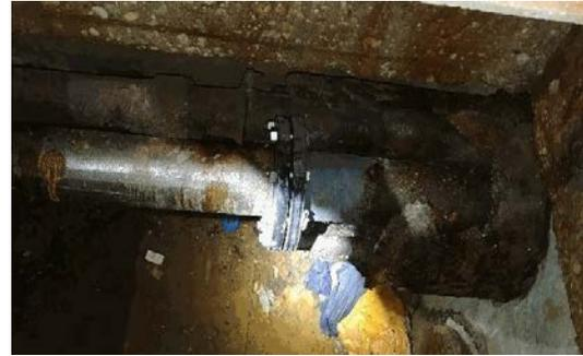
**Project Description** Replacement of existing Ricwil pipe in the scum concentration building at the Calumet WRP. The Ricwil pipe is a host pipe which contains steam, pumped condensate return, effluent water, and low pressure air piping.
