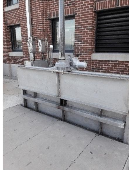
**Project Description** Replace seven beveled gear actuators with direct mount actuators at the O'Brien WRP's ultraviolet channel inlet gates.
