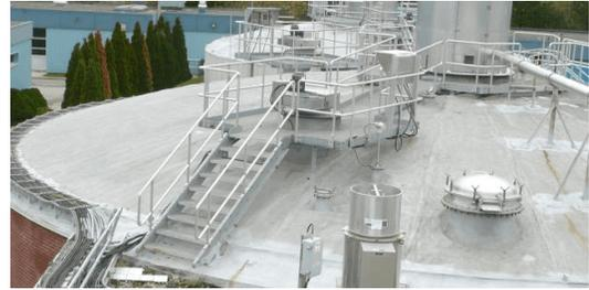
**Project Description** The work will remove all inorganic heavy solids which have accumulated and are not removable through the sludge draw-off system. The work will include rehabilitation of the digester covers and tank walls. Digester gas piping will be rehabilitated or replaced as required and the mixing system components will be rehabilitated to a working condition in Digesters 1 through 12. Also, the digester gas waste gas burners will be rehabilitated.
