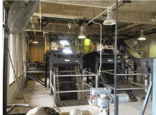
**Project Description** At the Hanover Park WRP, replace the grit classifier, two catenary fine screens with traveling bar rake screens, and the flat belt conveyor with an enclosed shaftless screw conveyor. At the Stickney WRP, replace two shafted screw conveyors for scum concentration with one shaftless screw conveyor and one shafted screw conveyor.
