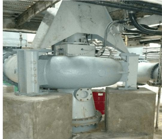
**Project Description** The purpose of this project is to rehabilitate Raw Sewage Pumps 1 and 2 at the Egan WRP. The work includes the replacement of the pump and motor bearings, seals, and related parts to restore the equipment to like-new condition. Also, two old-style centrifuge diverter gates will be replaced with slide gates furnished by the Maintenance & Operations Department. Hopper modifications will be made, as necessary, to allow for the installation of the diverter gates.
