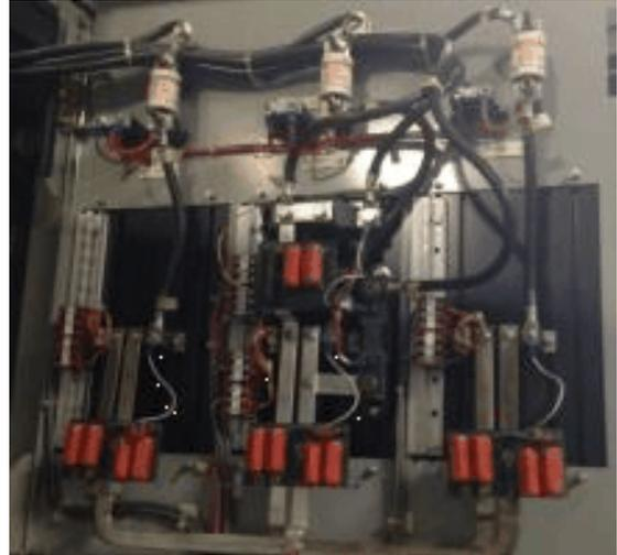
**Project Description** Furnish and deliver replacement excitation control equipment for the North Branch Pumping Station (NBPS) and Racine Avenue Pumping Station (RAPS) main sewage pump synchronous motors. Four new pump motor exciter control systems will be installed at both the NBPS and the RAPS. Installation will be performed by District trades under the direction of an excitation control manufacturer representative and the resident engineer.
