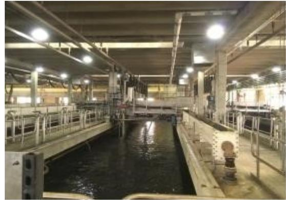
**Project Description** The scope of work includes the installation of seven aerated grit tank screw conveyor systems, the replacement of eight tank covers, and the demolition of eight bridge assemblies in the grit facility at the Calumet WRP.
