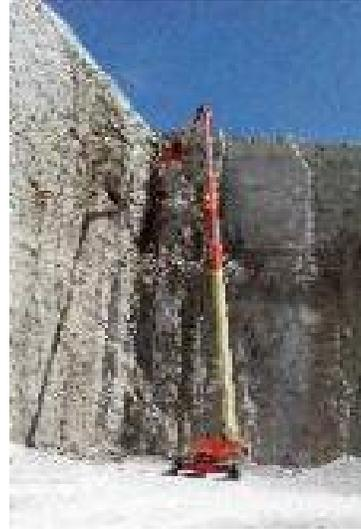
**Project Description** The scope of work consists of stabilizing the near-vertical excavated walls of the reservoir through the installation of rock bolts, rock dowels, cable bolts, chain link wire mesh, and shotcrete at locations where deemed necessary. Work will also include the installation of instrumentation and monitoring devices and related equipment.
