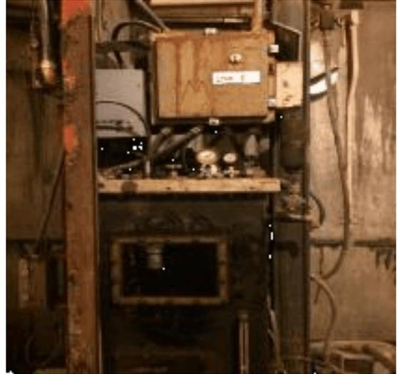
**Project Description** This project entails removing the existing hydraulic operator and accumulator assembly for Tunnel and Reservoir Plan Gate I at the O'Brien WRP and installing an electric actuator in its place. Five redundant hydraulic sluice gates will also be blocked open and decommissioned.
