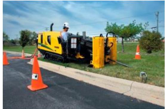
**Project Description** This project consists of the installation of 2,000 linear feet of six-inch diameter pressure pipe by directional drilling and the installation of air relief, blow off, and clean-out structures.
