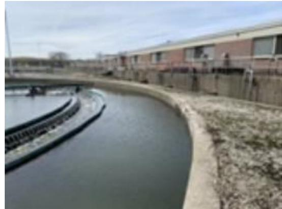
**Project Description** This project consists of concrete rehabilitation of Battery A final settling tanks at the Stickney WRP and rehabilitation of deteriorated and leaking roof deck and deteriorated concrete beams in the coarse screen room of the Racine Avenue Pumping Station (RAPS). This project will add steel railing and safety davit sleeves at final settling tanks and a permanent safety barrier along mixed liquor channel.
