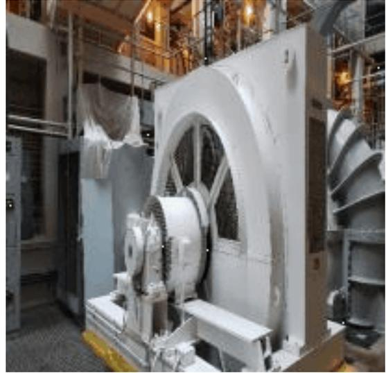
**Project Description** This project will rewind the motor stator and refurbish the rotor and exciter windings on main sewage pump motor No. 2 at the Stickney WRP.
