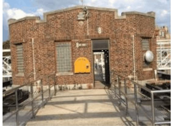
**Project Description** At gate houses No. 1 and 2, perform tuckpointing, restore the glass block and parapet, and remove and replace the roof. Similar restoration work must also be performed at the sludge concentration building.
