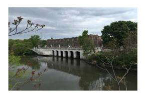
**Project Description:** Provide grouted fiberglass fiber reinforced plastic jackets around the existing concrete columns to protect columns from erosion. Repair underwater deteriorated concrete of the east wall and under the deck wall. Repair deteriorated concrete stairs and concrete deck. Restore balustrade and deck lighting.
