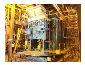
**Project Description:** This project will furnish, deliver, and install controls, programming, and other required appurtenances to provide a co-fire implementation of Boilers 3, 4, 5, and 7 using natural gas and digester gas through existing gas trains. Use of co-fire logic and technology shall enable full utilization of available digester gas produced at the plant. Controls for Boilers 1 and 2 will be upgraded as well.
