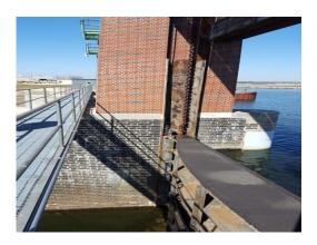
**<u>Project Description:</u>** The purpose of the project is to furnish and deliver a cofferdam to assist District trades with the rehabilitation of Gate 5 at the Lockport Powerhouse.
