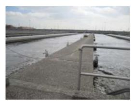
**<u>Project Description</u>**: Install safety railings around aeration tanks, preliminary settling tanks, contact chambers, and final settling tanks for worker safety and to meet Occupational Safety and Health Administration regulations.
