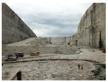
The first section of the McCook Reservoir, holding 3.5 billion gallons, is nearing completion in 2017. The reservoir is the final component of the Metropolitan Water Reclamation District of Greater Chicago's Tunnel and Reservoir Plan.
