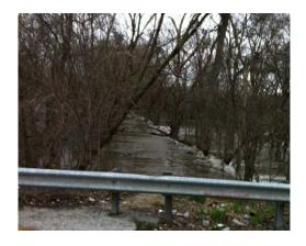
**Project Description:** The Lyons Levee is located on the east bank of the Des Plaines River and is approximately 4,000 feet long, beginning at Joliet Road at the upstream end and extending approximately 700 feet downstream of 47th Street. The scope of the project involves the restoration and improvement of the levee to a condition that will elevate the levee to modern design standards, provide flood protection, and prevent overtopping by events up to a 100-year design flood.
