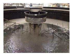
**Project Description:** This project will convert two of the new gravity concentration tanks (GCTs) into fermenters and install a pumping station to pump the fermentate directly into the West Side primary effluent conduit feeding the secondary aeration batteries. This project will also install a gas detection system for the new gravity concentration tank building.
