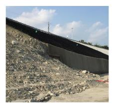
**Project Description:** The scope of work consists of constructing approximately 2,000 linear feet of a soil nail retaining wall along the western and southern sides as well as slope stabilization work around the entire perimeter of Expanded Stage 2 of the McCook Reservoir.
