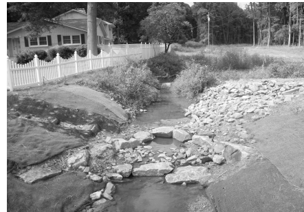
Rock cross vane installation on Muddy Creek.
