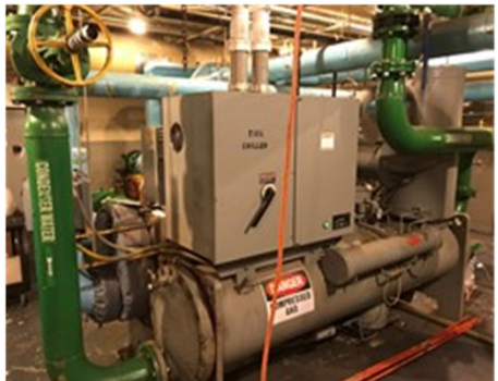
Replace Chiller at MOB
