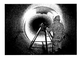
Project Description: This project consists of the rehabilitation of 810 feet of 6'x7' semi-elliptic cast-in-place concrete sewer and inlet/outlet structures. The Summit Conduit begins on the northwest side of the Des Plaines River and extends southeast under the Des Plaines River and the Stevenson Expressway to the northwest side of the Chicago Sanitary and Ship Canal.
