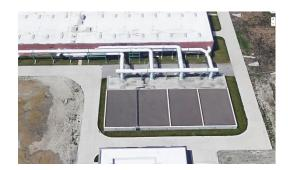
**Project Description:** Three biofilter facilities will be constructed, one for sludge concentration and overhead weir, one for the southwest coarse screen, and one for the post-centrifuge building. The facilities will include new biofilters, Heating, Ventilation, and Air Conditioning equipment, ductwork, and other ancillary equipment.
