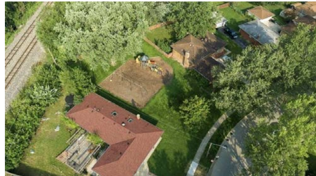
The North Creek Flood Relief Project, funded by the District at a cost of $1.6 million, involved constructing a new culvert for North Creek to alleviate flooding and safeguard 56 residential structures in the vicinity of Flanagan Park.
