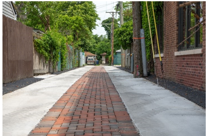
According to the District's Green Infrastructure Partnership Program, permeable alleys are more attractive and hold more stormwater. The District and municipal partners completed several green alley projects, as shown above in Maywood.
