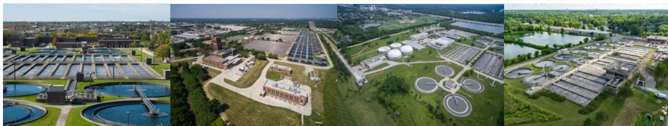
Kirie, O'Brien, Egan, and Hanover Park WRPs are four of seven wastewater treatment facilities that comprise the North Service Area with regulatory permit requirements for phosphorus limits coming online in the new future.
