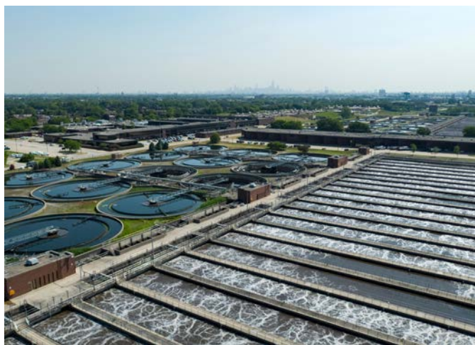
The Stickney Water Reclamation Plant (WRP) is one of the largest wastewater treatment facilities in the world. It serves residents in the central part of Chicago and 46 other communities within a 260-square-mile area. The Stickney WRP consists of two plants: the original West Side Plant, which was placed in service in 1930, and the Southwest Plant, which was placed in service in 1939.
