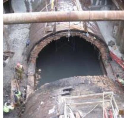
**Project Description** This project will rehabilitate a portion of the 100+ year-old conduit lying under 39th Street (Pershing Road), stretching from a former pumping station near Lake Michigan to its discharge at the Racine Avenue Pumping Station (RAPS). The project includes approximately 3,280 feet of concrete intercepting sewer rehabilitation from Halsted Street to RAPS, as well as associated manholes and connecting structures.
