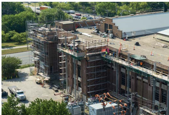
Steel spandrel beams are rehabilitated for the pump and blower house at the O'Brien Water Reclamation Plant.
