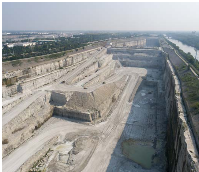
Excavation work progresses at the McCook Reservoir in the summer of 2025. When complete, the total storage capacity at the reservoir will be 10 billion gallons.
